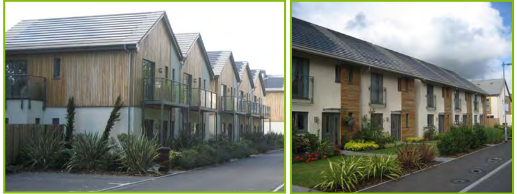
Solar panels and edible gardens in Graylingwell Park, Chichester
