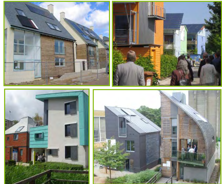
Top left: Solar panels on new homes in Upton, Northampton
